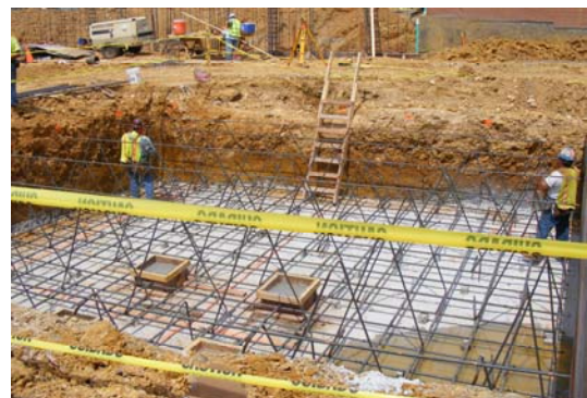
FIGURE 10: Neat Cut Footings
