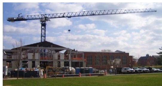
FIGURE 6: Tower Crane for New Centennial
