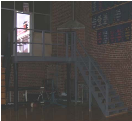
FIGURE 4: Temporary Interior Stair Tower
