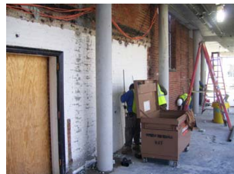
FIGURE 2: Circular Columns Along North Wall
