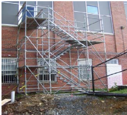
FIGURE 3: Temporary Exterior Stair Tower
